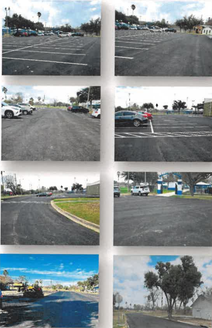
Lion's Park Paving Project
