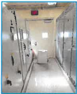
AJC Repair MCC Room
