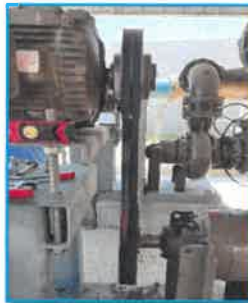
RAS Pump Belt Repair
