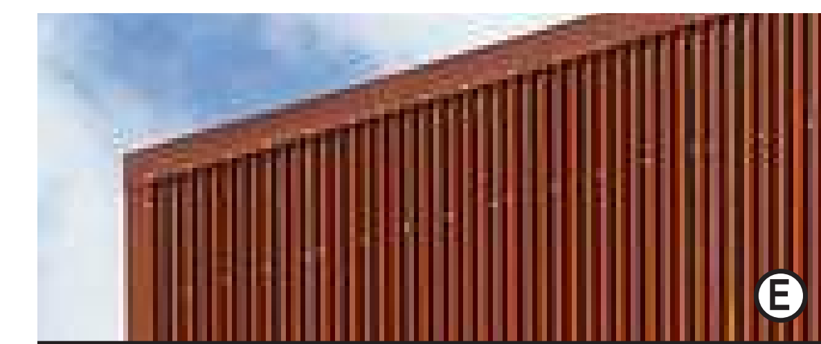
E CORRUGATED METAL SIDING - OXIDIZED
