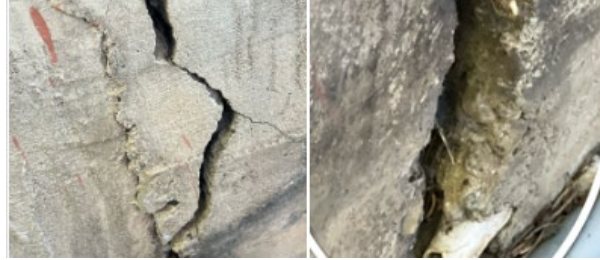
(Detail 9) Cracking Foundation.
