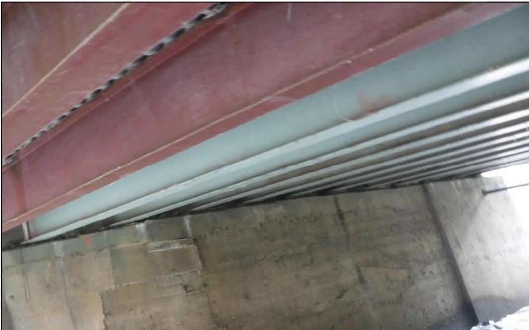
Superstructure looking north.
