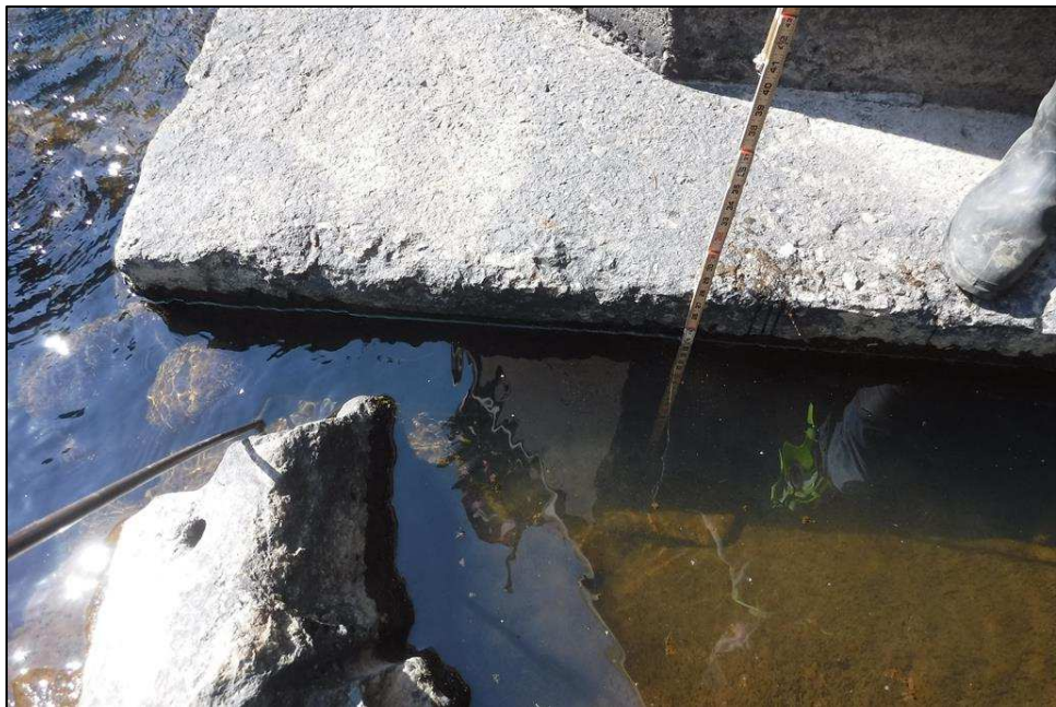
P4 northwest corner exposed footing.
