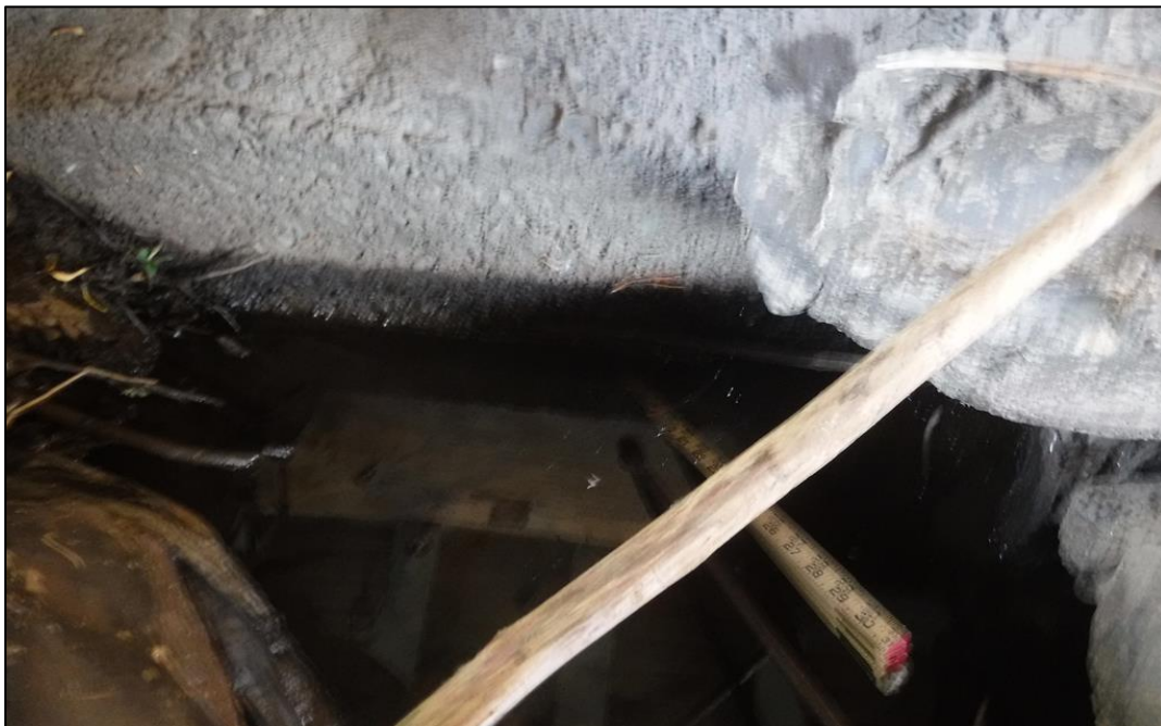
Abutment 5 undermining.
