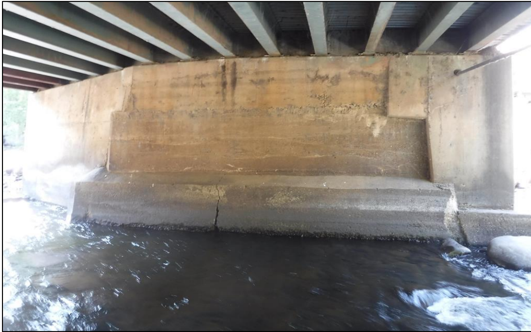
General view of Pier 3.
