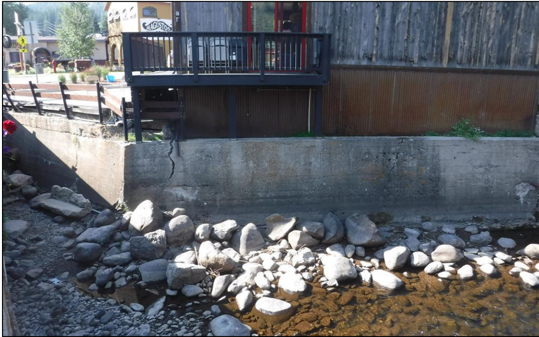
View of SW retention wall.
