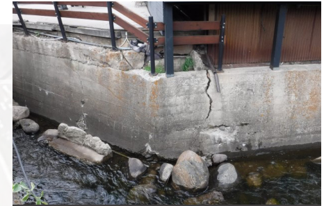
B Existing Wall Crack and undermining adjacent to bridge and below Minturn Anglers Fly Shop Structure
