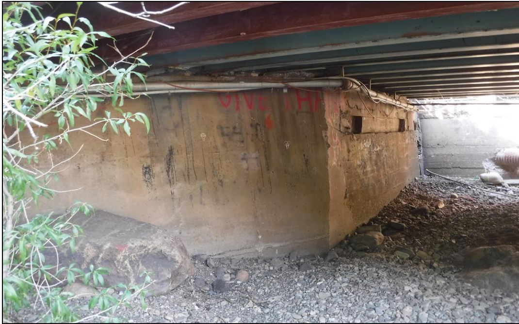
General view of Abutment 1.
