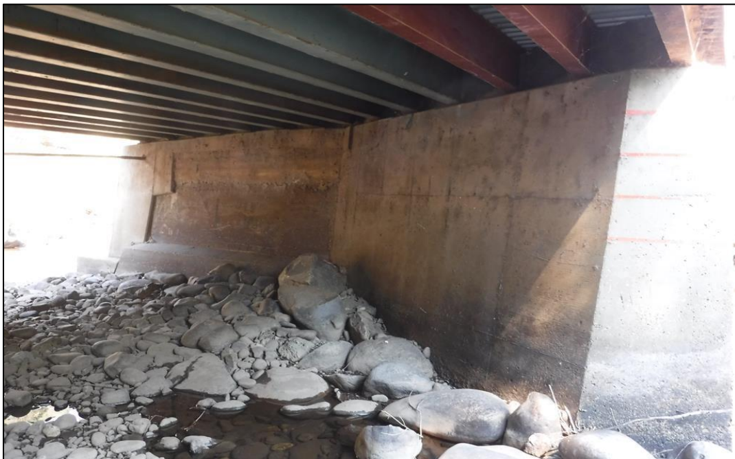
General view of Pier 2.
