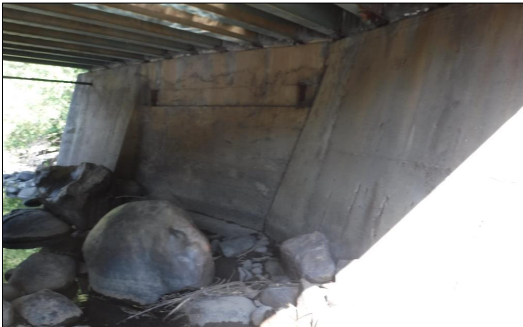
General view of Abutment 5.
