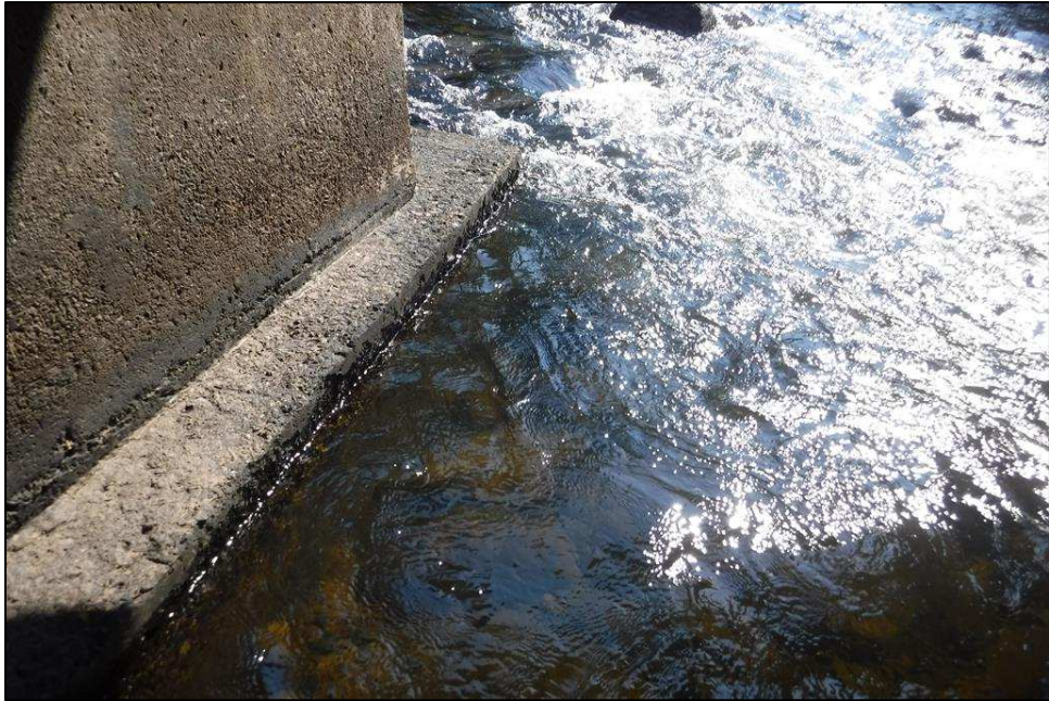
P4 south side exposed footing.
