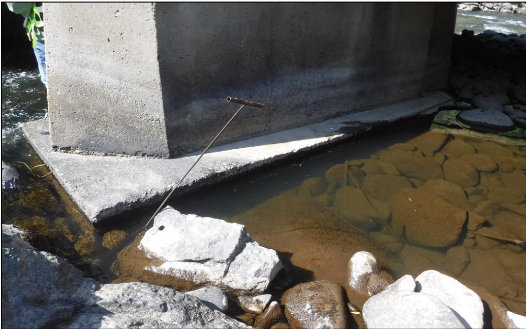
P4 exposed footing at north side.
