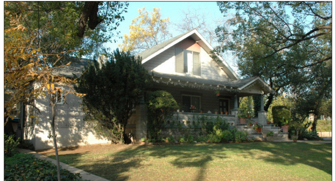
Above: House-form buildings with large yards shape the streetscapes.
