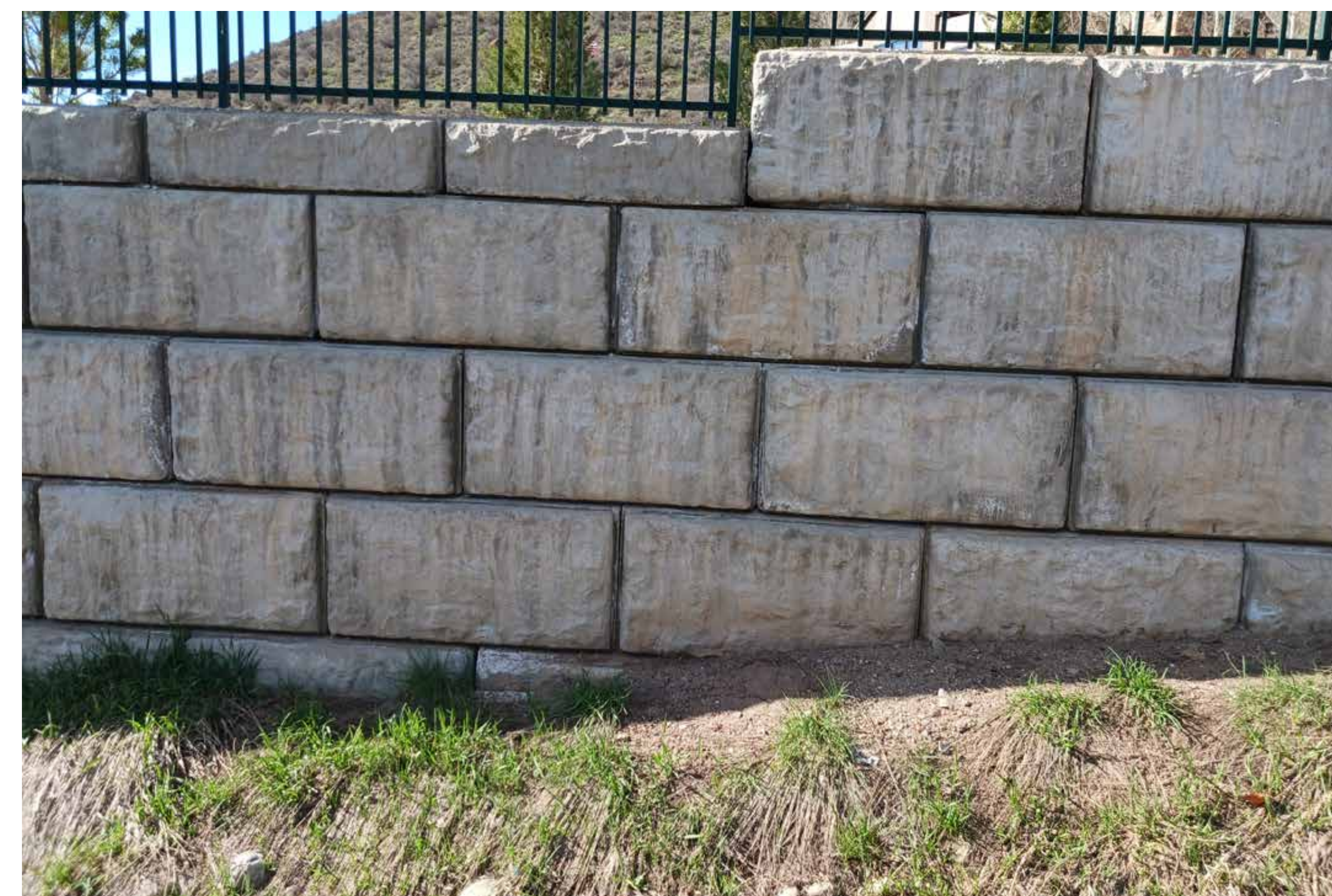
Existing Concrete Block Wall
