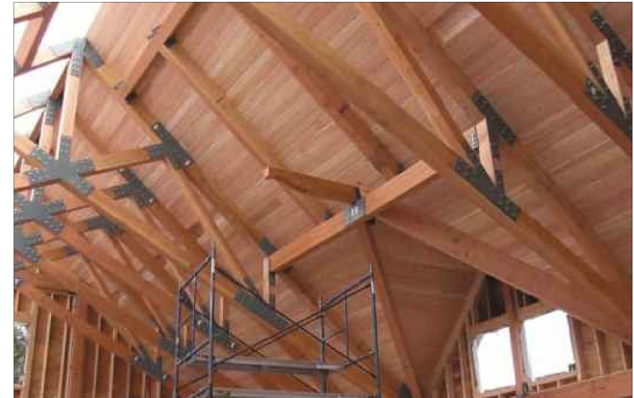
HEAVY TIMBERS WITH STEEL PLATES AND BOLTS
