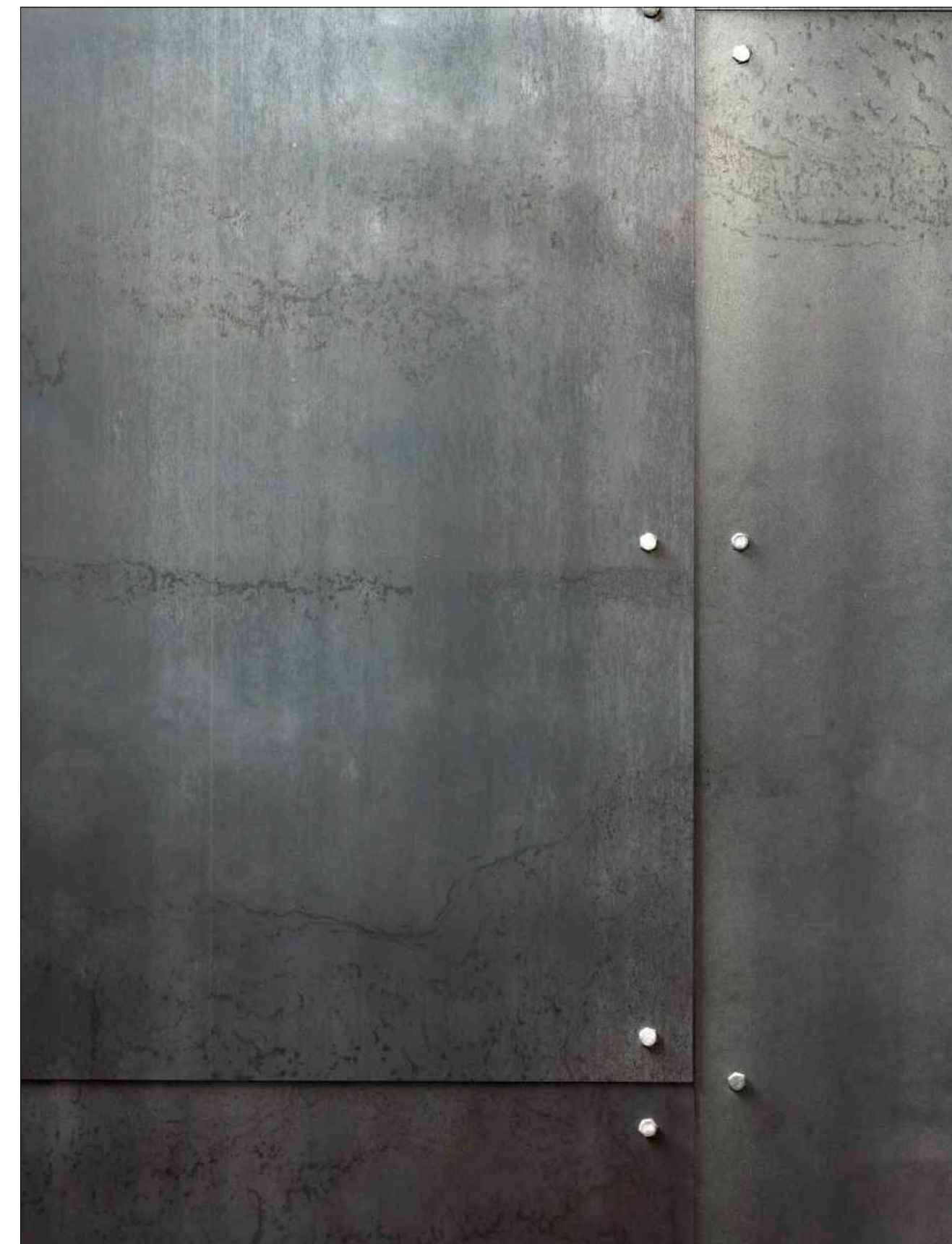
BLACKENED STEEL. TO BE USED AT GARAGE DOOR, FLASHING, MULLION CAPS, AND COLUMNS.
