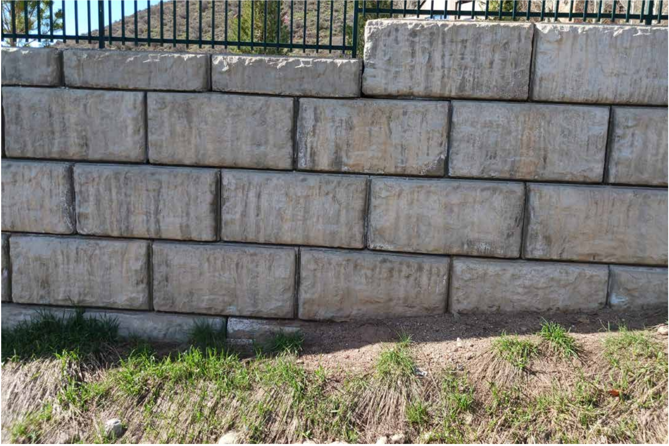
Existing Concrete Block Wall
