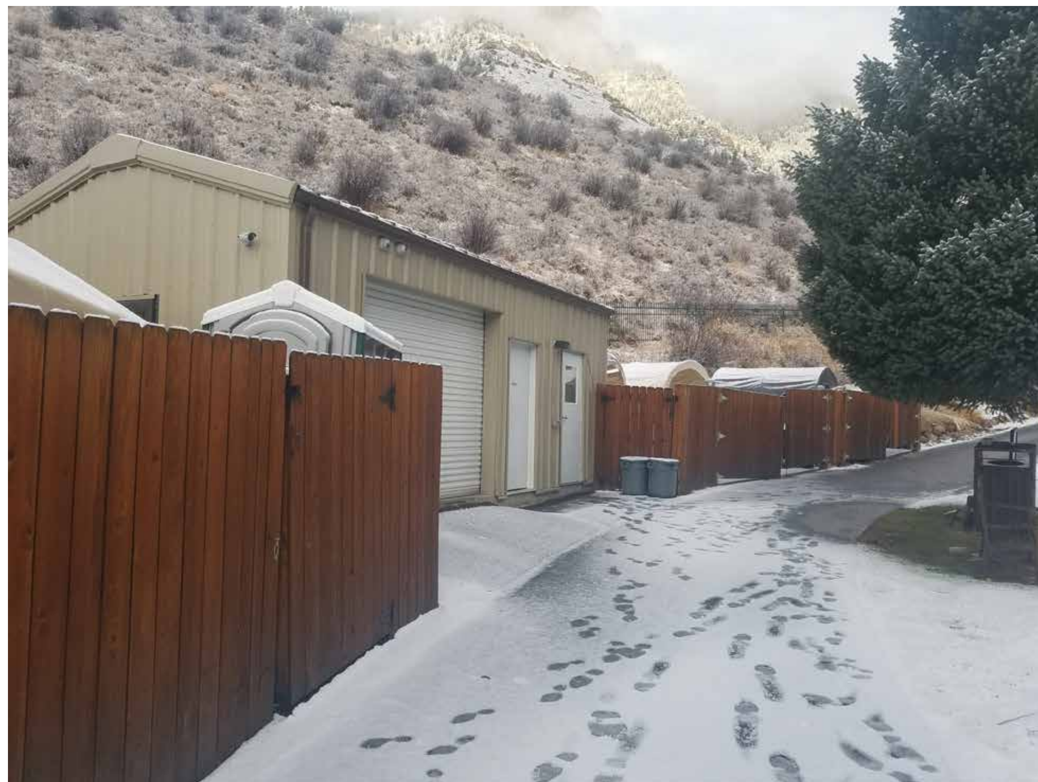
Existing maintenance building
