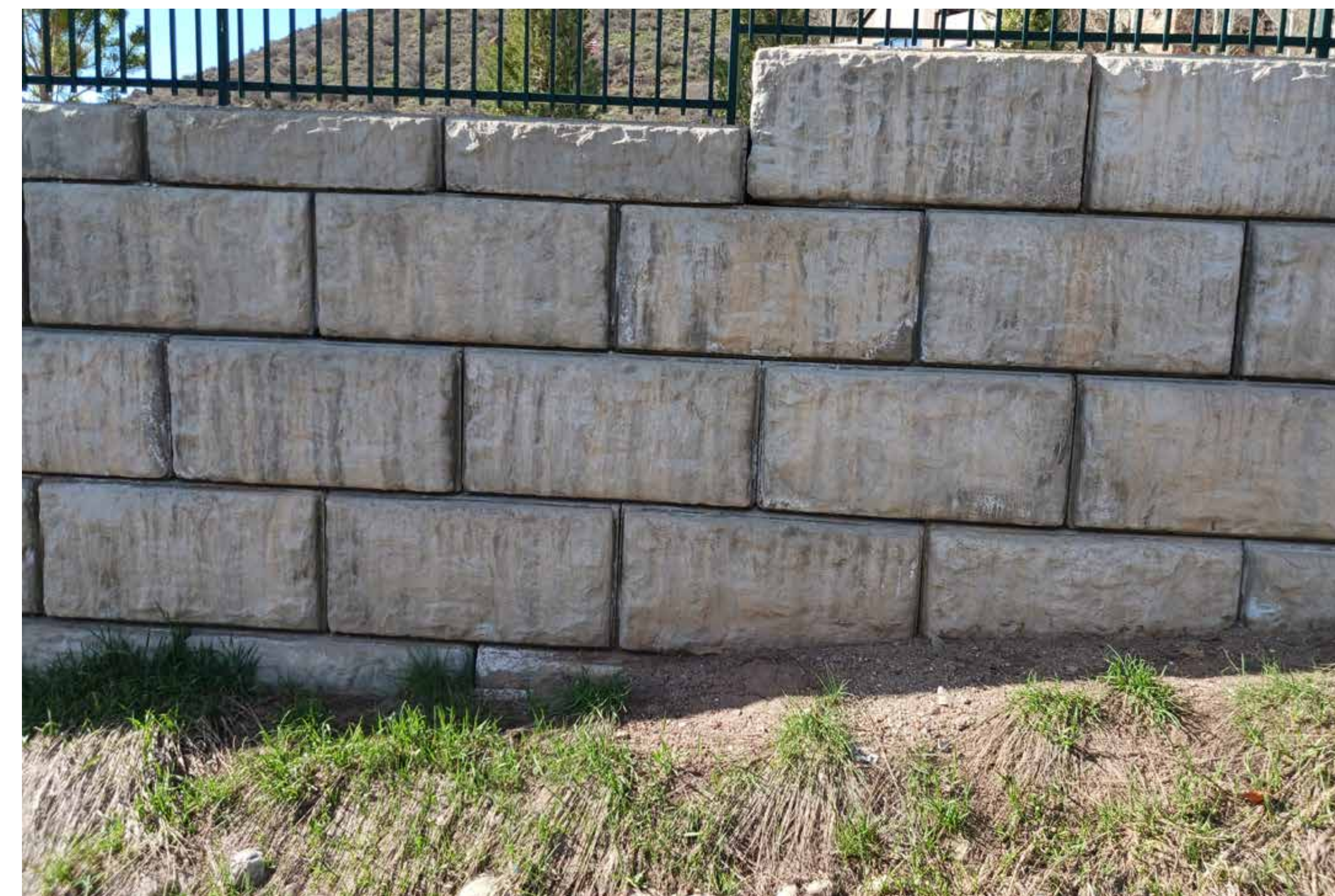
Existing Concrete Block Wall
