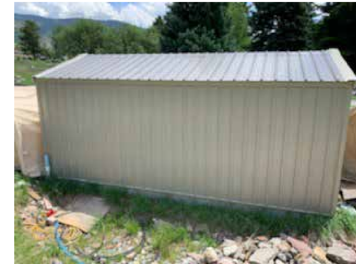
Existing Maintenance Building
