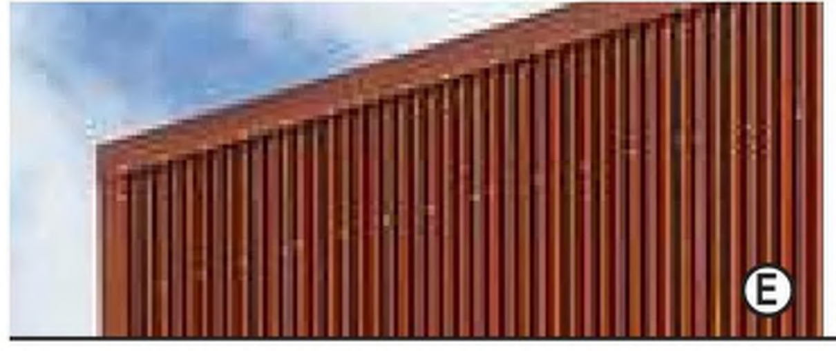
E CORRUGATED METAL SIDING - OXIDIZED
