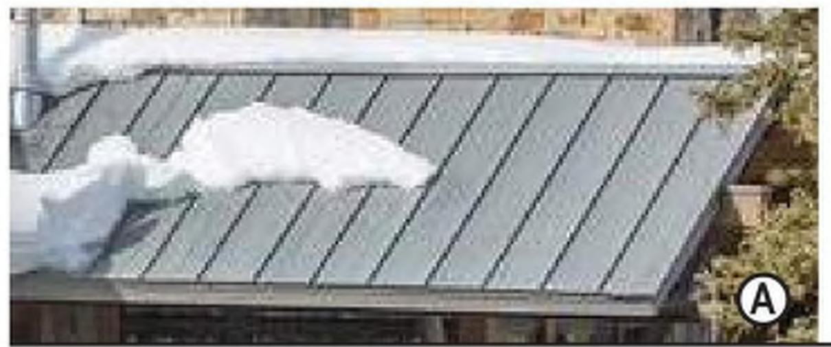
A STANDING SEAM METAL ROOF - GREY
