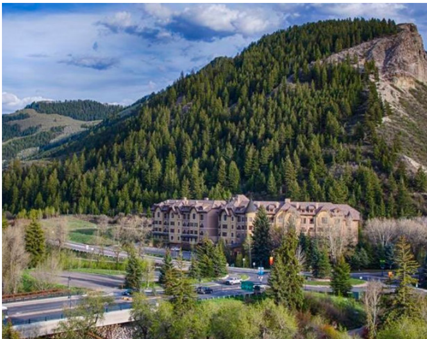
Photo courtesy of Uncover Colorado
