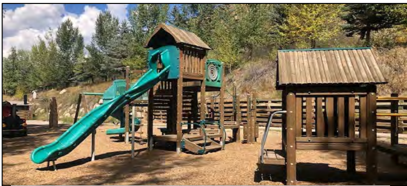
Non-Code Compliant Playground Structure
