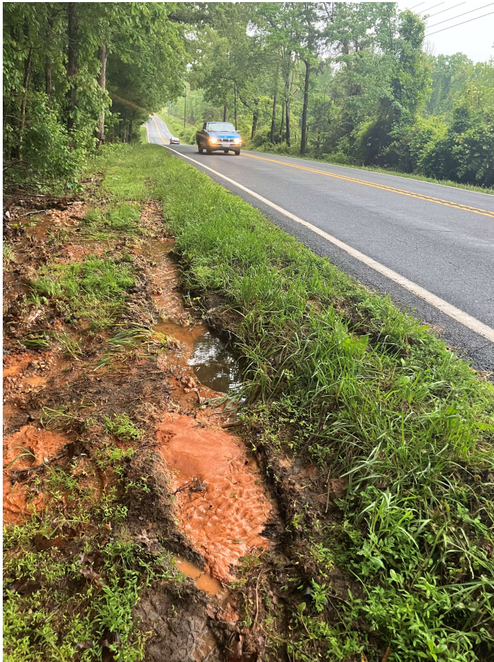
Figure 3. Break site. Appears to be tire tracks over pipe location
