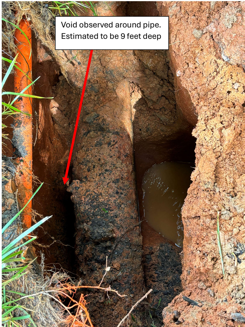
Figure 4. Exposed water main at break site
