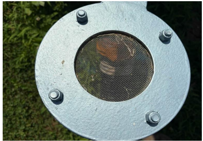
Overflow Pipe Screen
