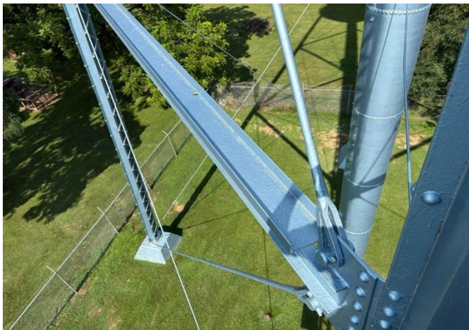
Strut and Rod Connections
