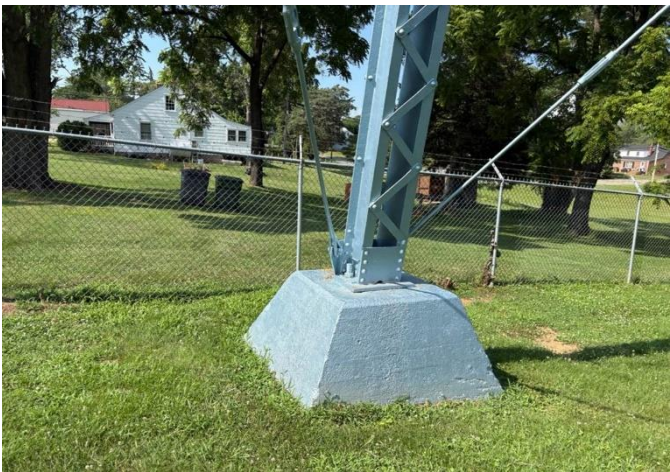
Foundation, Anchor Bolt, and Rod Connection
