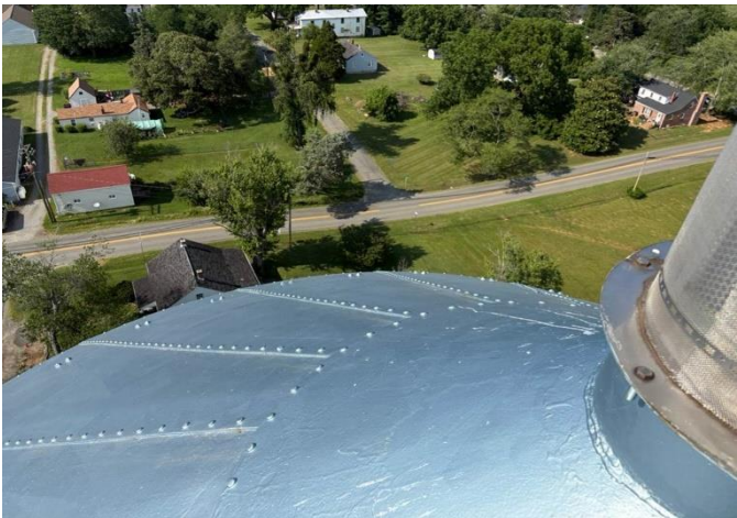
Exterior Roof Coating
