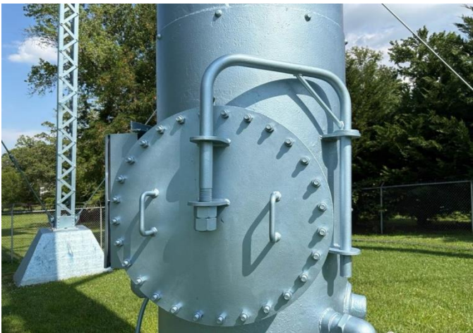
Multi Bolt Riser Manway with Davit Arm
