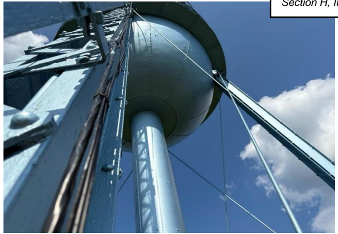
Exterior Bowl and Riser Coating
