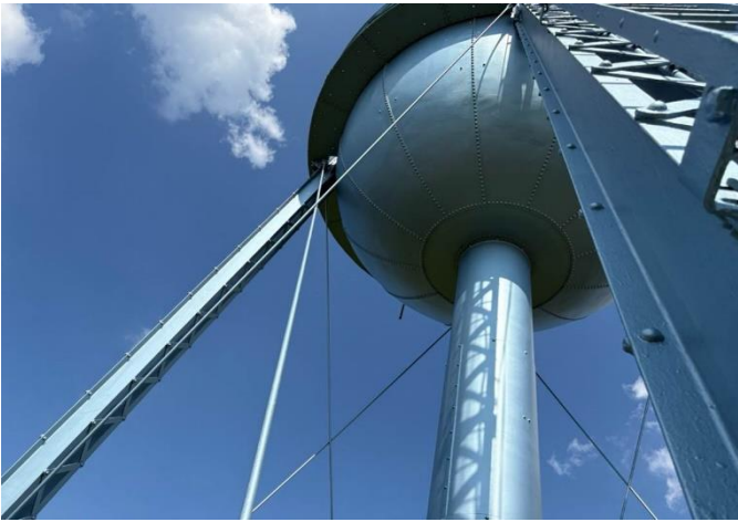
Exterior Bowl and Riser Coating
