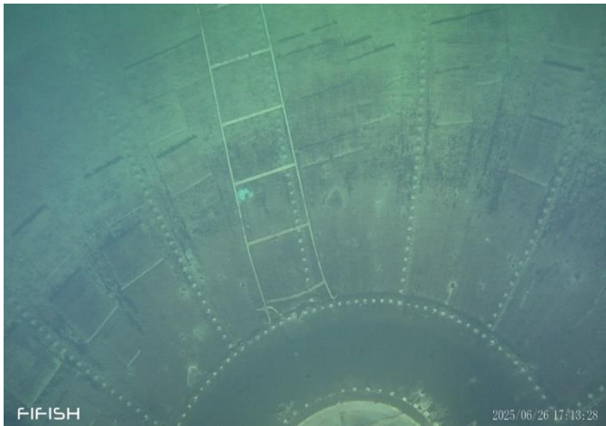
ROV Sidewall and Bowl Coating
