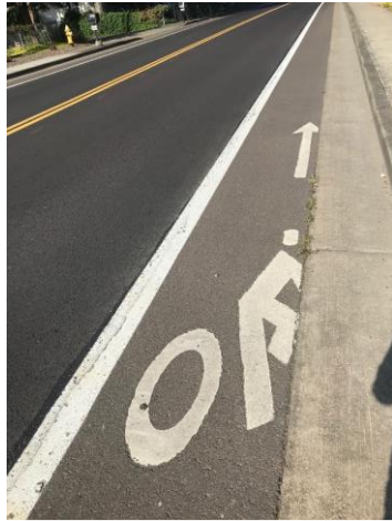
Thermoplastic Bike Lane symbol Millersburg Drive, 12 years old
