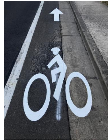
New Thermoplastic Bike Lane symbol
