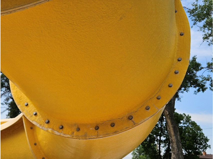
Figure 7: Cracked flange on waterslide.
