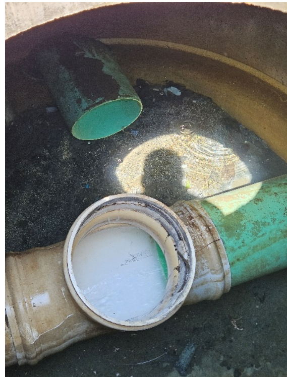
Figure 4: Strainer manhole after standpipe removed.
