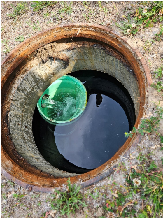
Figure 3: Strainer manhole full of water with standpipe.
