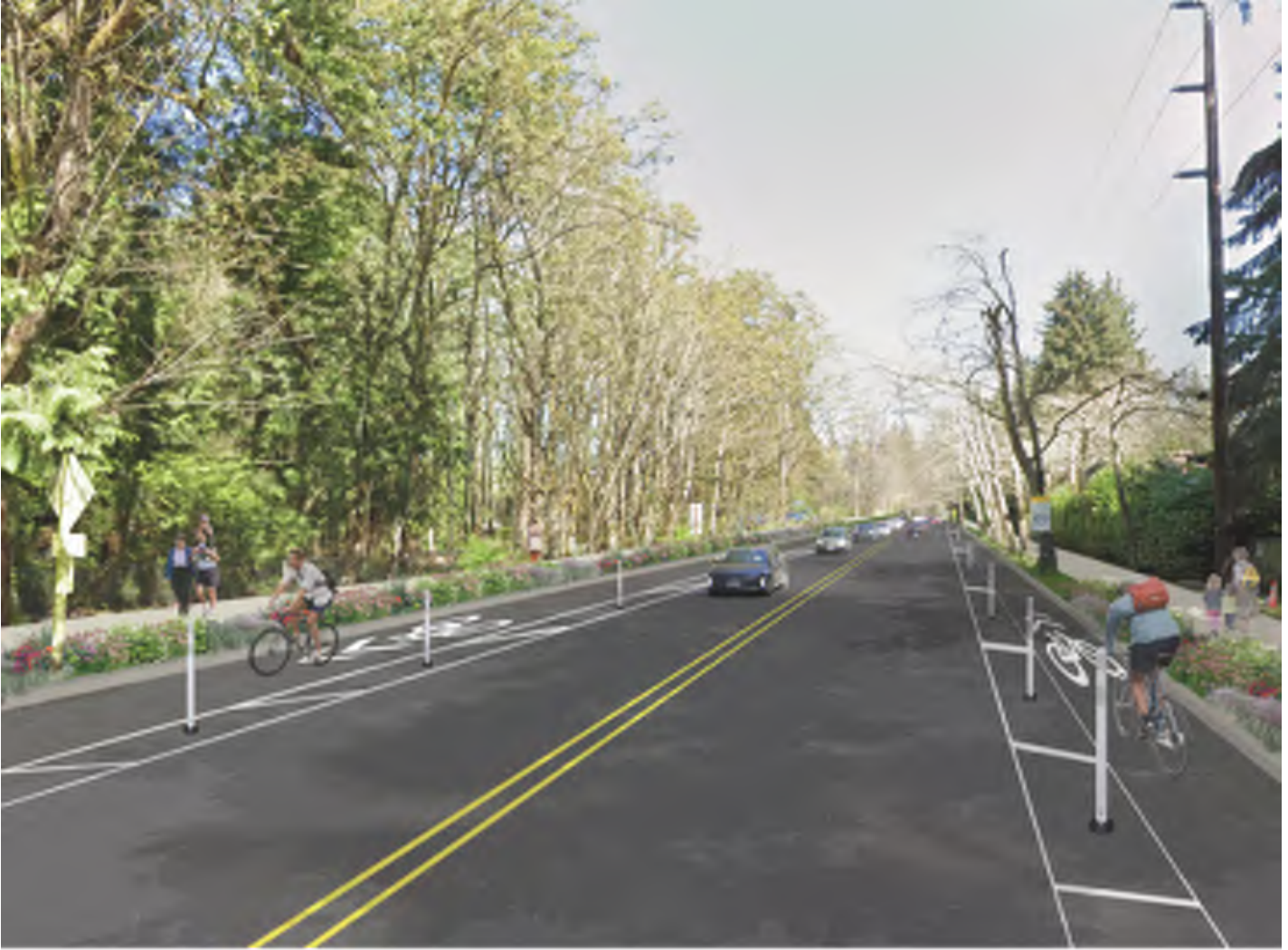
Figure 1: Separated Bike Lane
