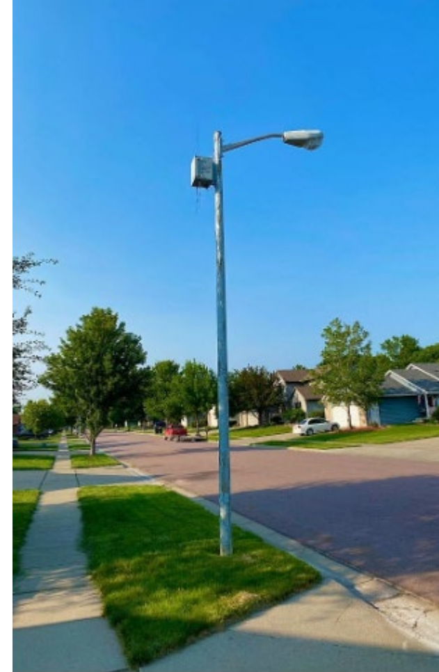
Example of small antenna on light post
