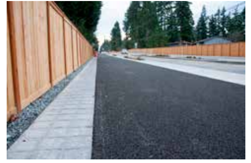
Scored pavement treatment
