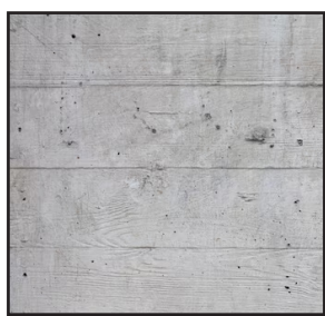
6 CONCRETE BOARD FORMED
