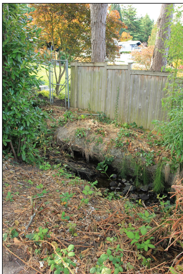
Stormwater channel incision and undermined bank. Note proximity to property boundary.
