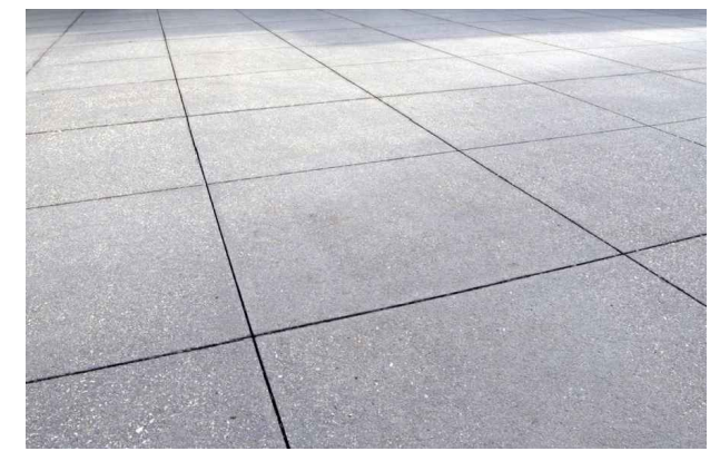
SAWCUT CONCRETE EXAMPLE
