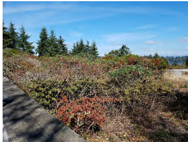
WSDOT Maintenance building rooftop – shrub mass along back wall.
