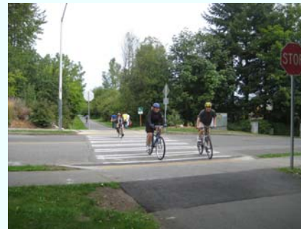
Per guidance in the 2012 AASHTO Bike Guide, Seattle is phasing out bollards and using other designs to enhance safety at roadway/trail crossings (Burke Gilman Trail).
