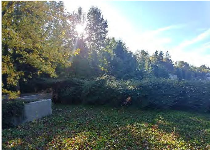
Photo 16. English ivy along bridge deck. Tree planter to the left has ample space for maintenance.
