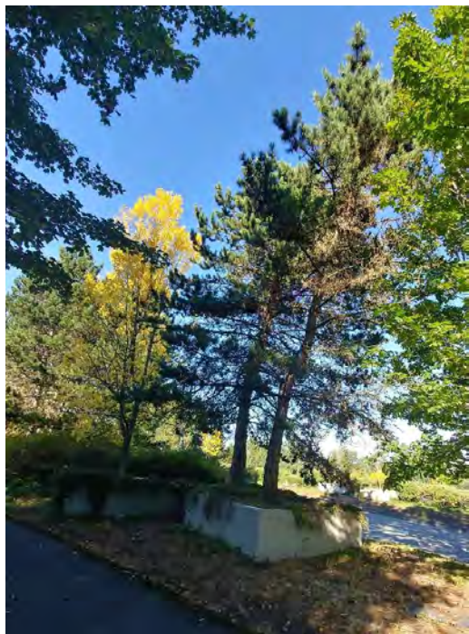
Photo 17. Trees in planter boxed require pruning. Some with uncorrected leans will require replacement.
