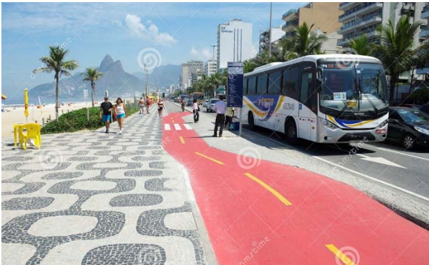
Figure 2. Example showing colored/textured pavement used to demarcate bike and pedestrian travel ways (Brazil)
