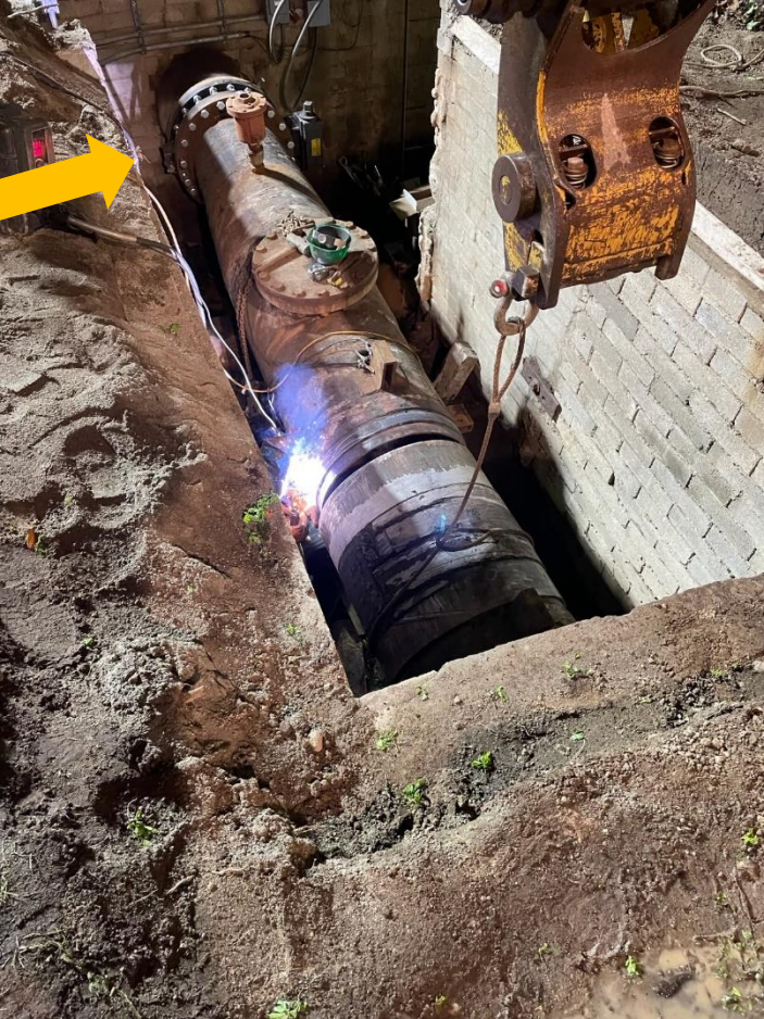
Replacement 24-in butterfly valve in place and piping welded back together
