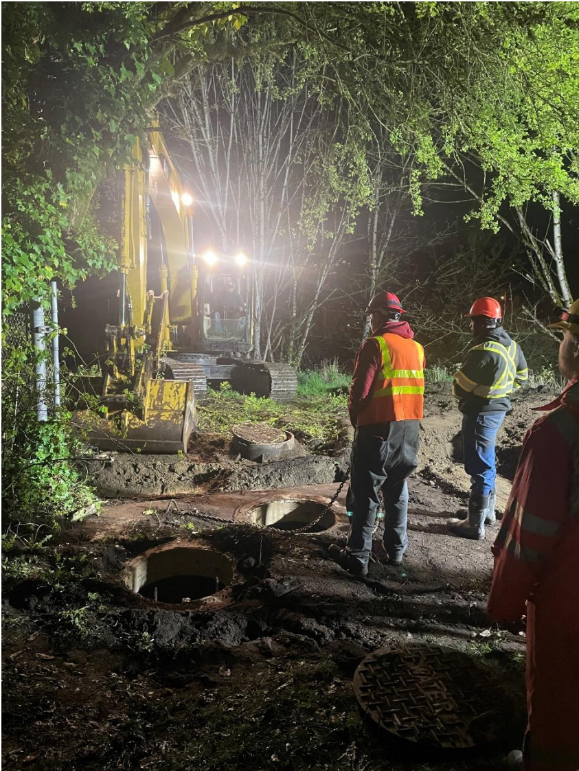
Valve vault before excavation
