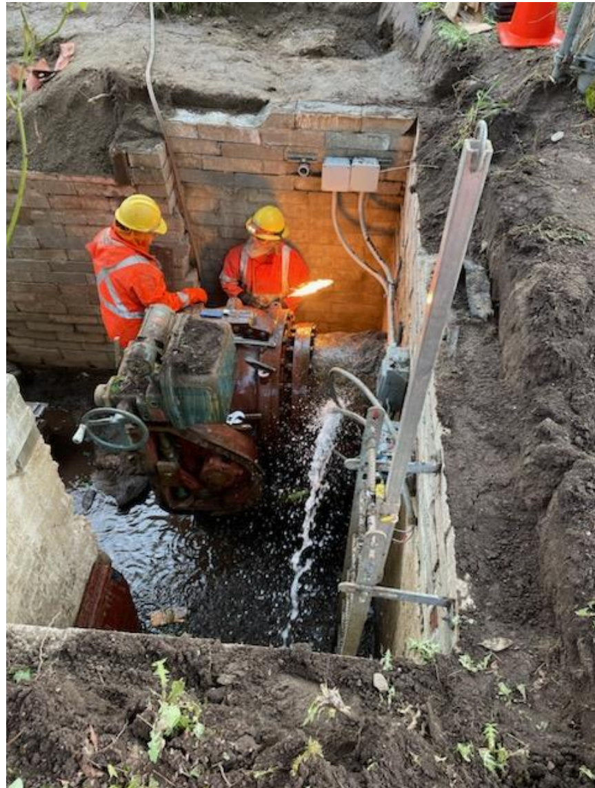
Removing 24-in ball valve
