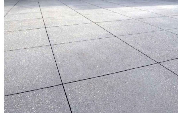
SCORED OR SAWCUT CONCRETE EXAMPLE
