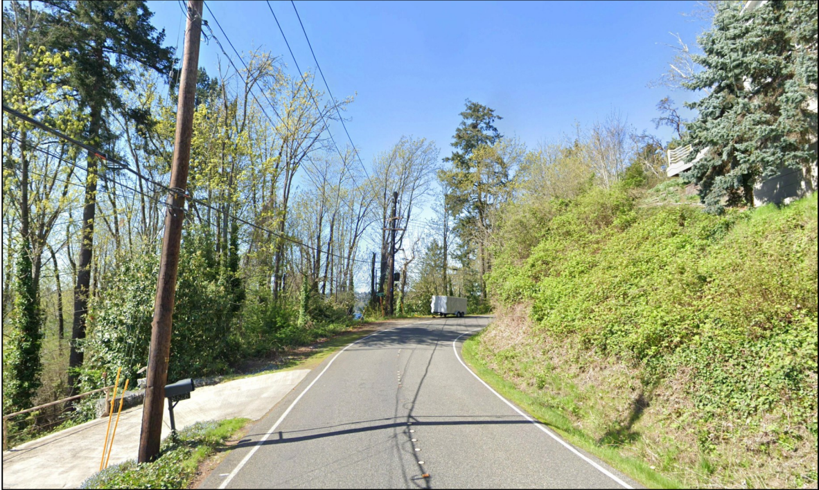
Photo of existing poles at West Mercer Way and East Mercer Way
