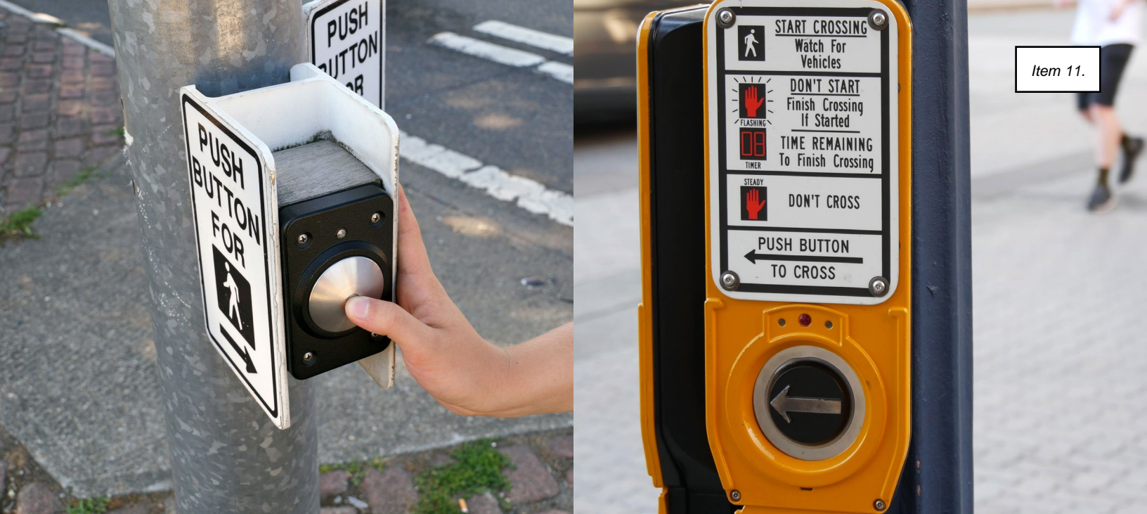
Figure 2-17 “H-style” (left) and APS-style pedestrian pushbutton (right)
