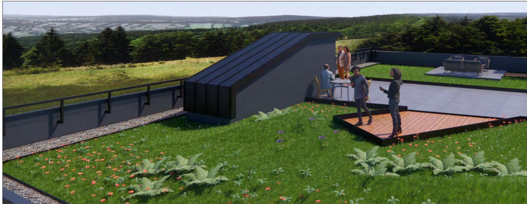
EXISTING PARAPET EXISTING HEIGHT IS BELOW 42" REQUIRED.
