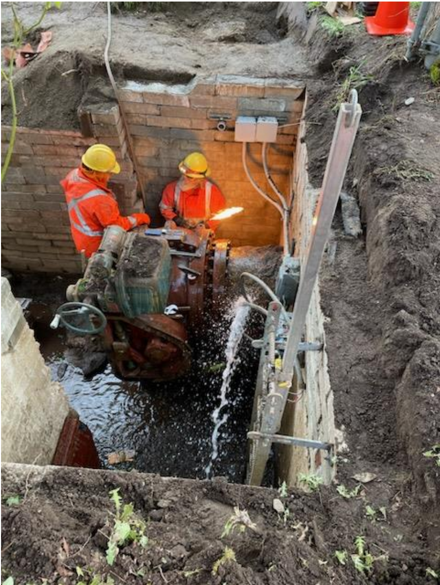
Removing 24-in ball valve
