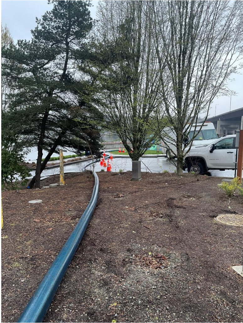
Bypass pumping setup from Bellevue Enatai to Mercer Island
