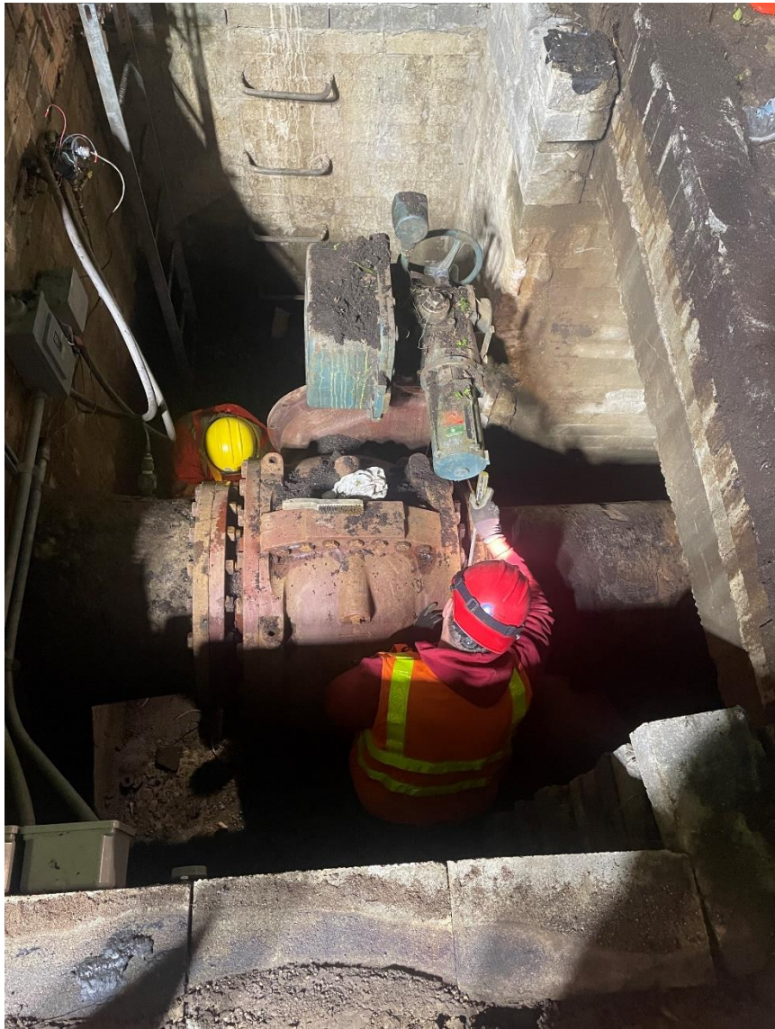
24-in ball valve that stuck closed
