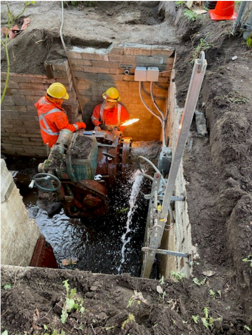
Removing 24-in ball valve
