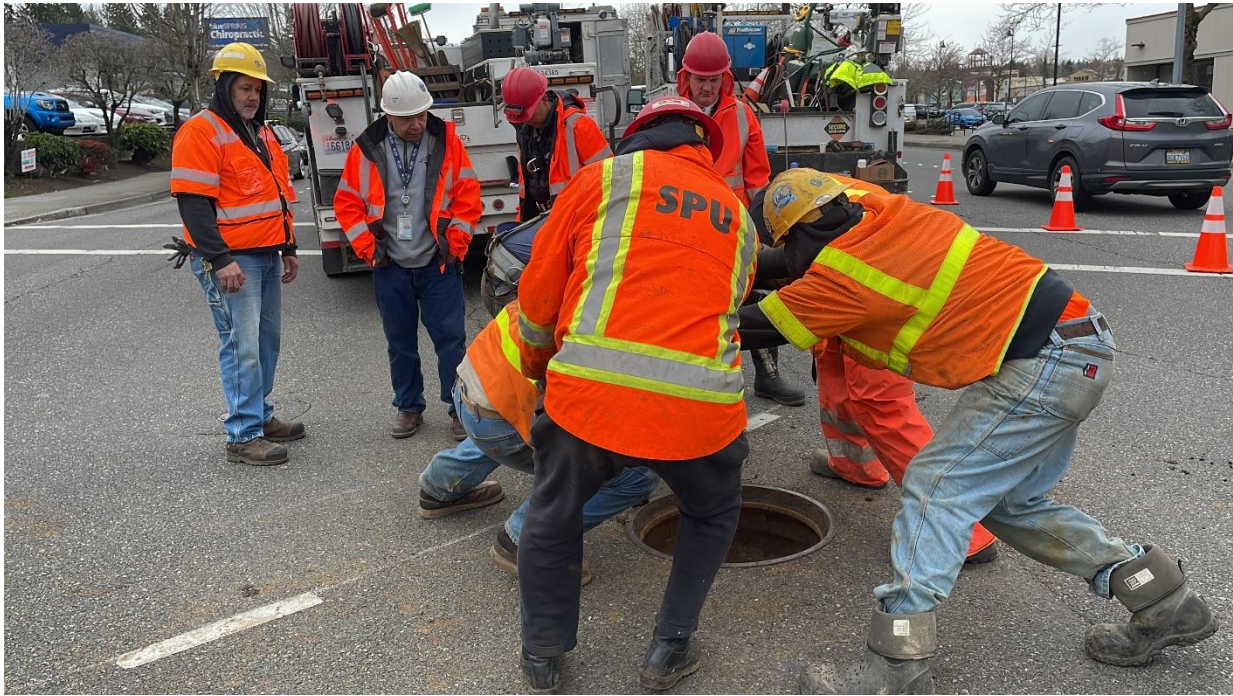
Crews manually turning the valve using a t-wrench attached to the top valve gear
