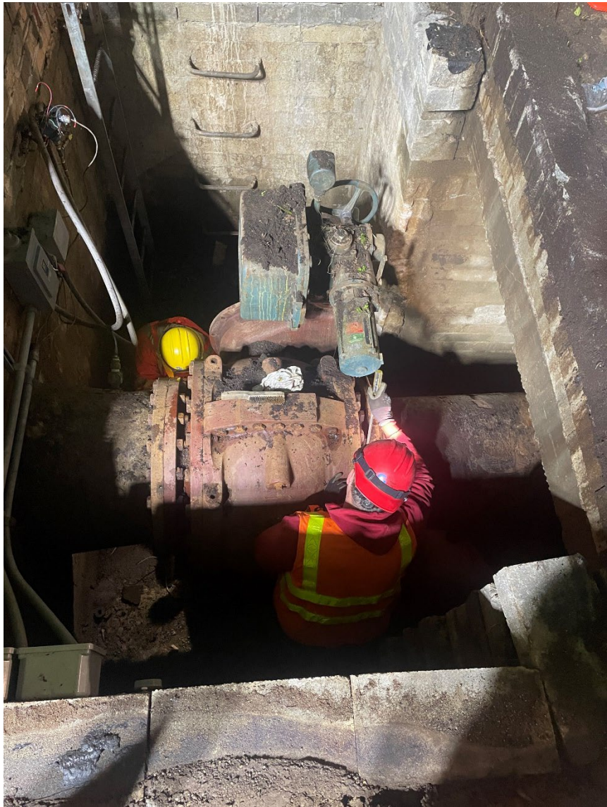
24-in ball valve that stuck closed
