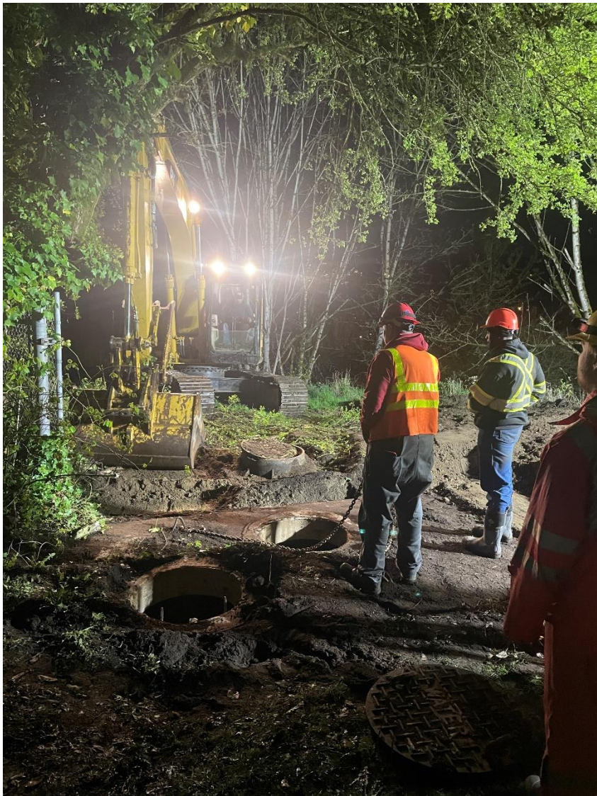
Valve vault before excavation
