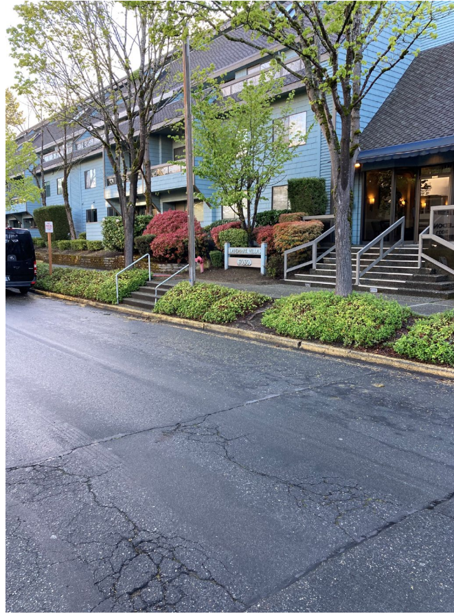
Existing sidewalk is much higher than existing street
