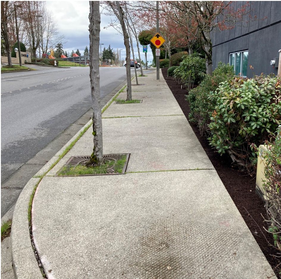
Existing trees in poor health due to limited growing area
