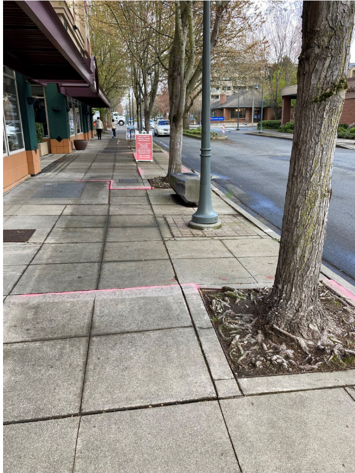
Uneven sidewalk panels, high root masses
