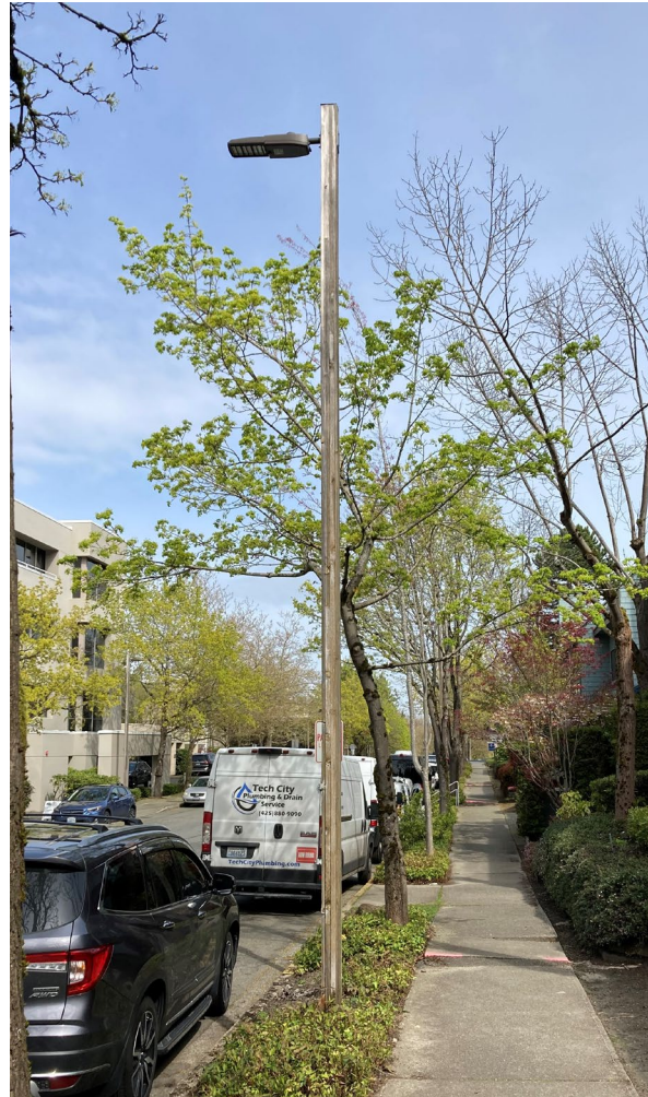
Typical wood pole to be replaced
