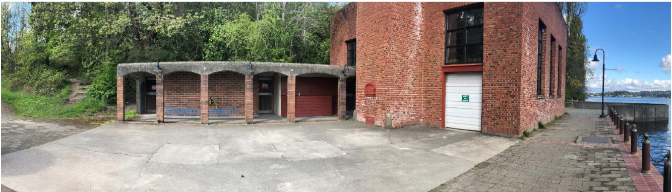
Figure 3: existing waterfront plaza with the boiler building on the right and restrooms on the left
