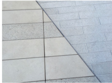
A Unit Pavers on Grade
