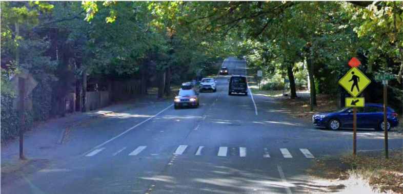
Photo C: Marked crossing at SE 63rd Street with signing (facing southbound).
