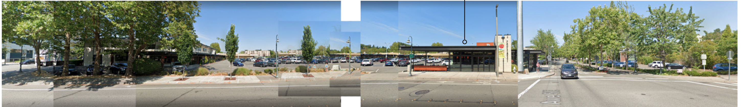
SE 32ND ST. LOOKING NORTH TOWARDS SITE
