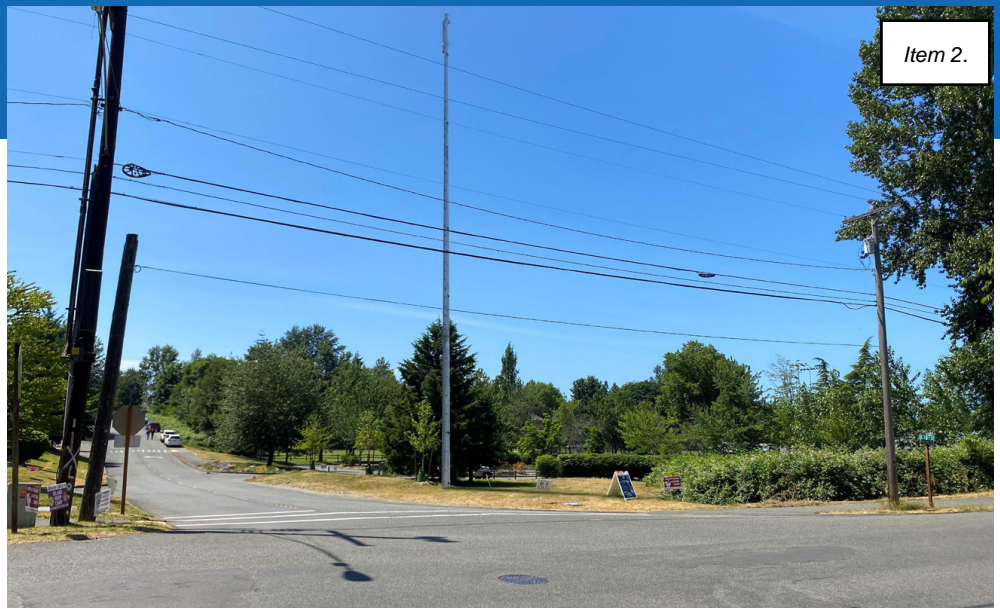
Rendering of proposed data collection equipment on a new 80-foot pole near South Mercer Playfields.
