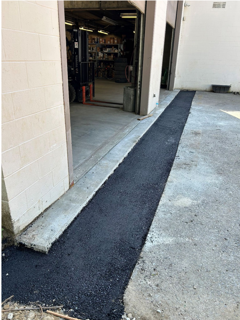
AB6901 | EXHIBIT 2 | GRADE BEAM COMPLETE AT MECHANIC GARAGE DOORS
