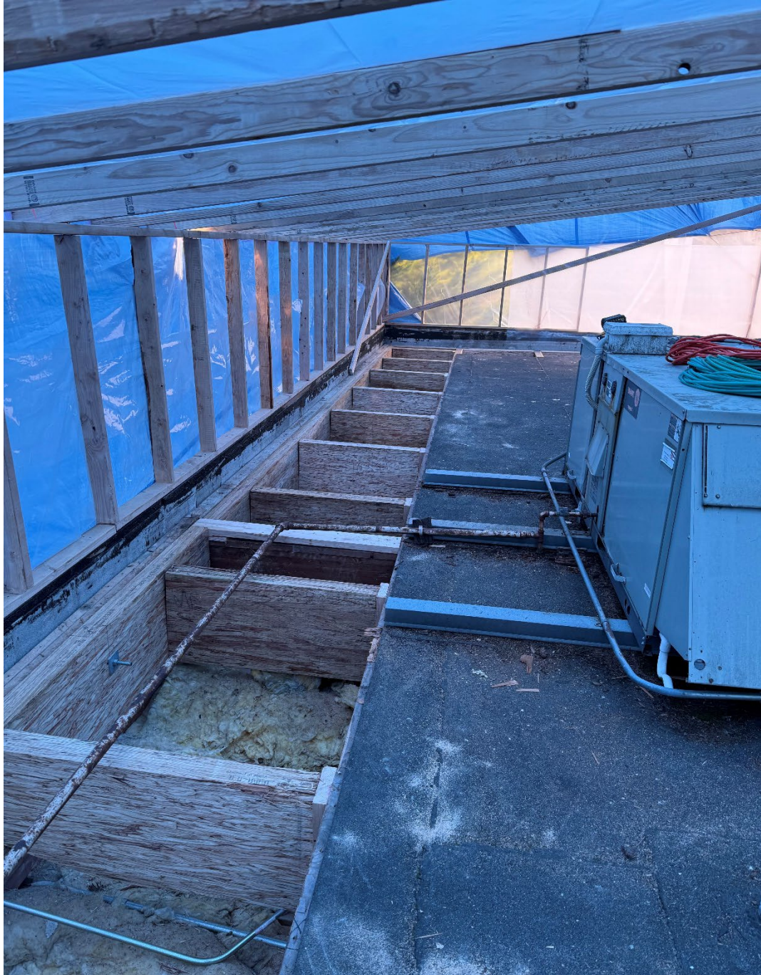
AB6901 | EXHIBIT 2 | UPPER ROOF REINFORCEMENT
