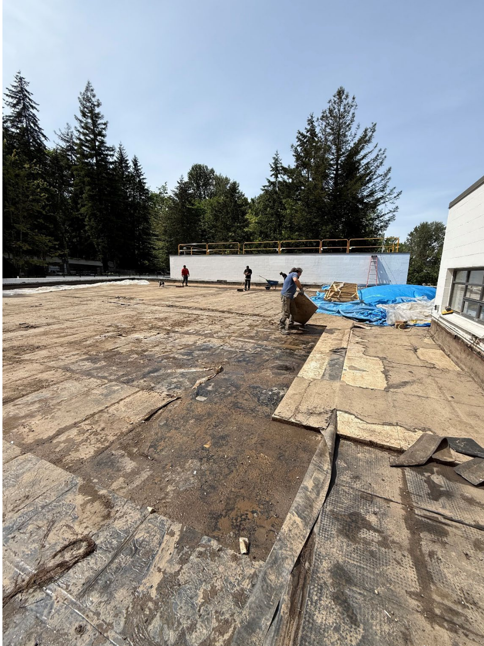
AB6901 | EXHIBIT 2 | GREEN ROOF ASSEMBLY REMOVAL
