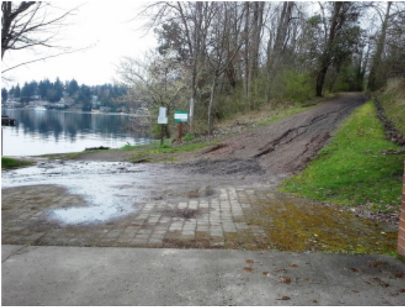
Photo 3A – Gravel maintenance road
