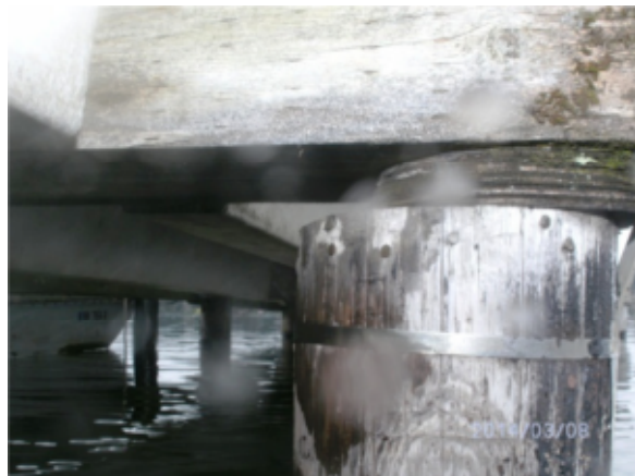
Photo 18A – Plywood shims between cap and pile
