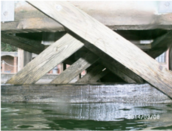
Photo 19A – Diagonal bracing
