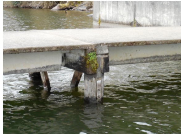
Photo 8A – Typical pier construction
