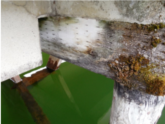
Photo 13A – Treated cap beam at pile
