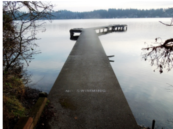
Photo 22A – Small pier
