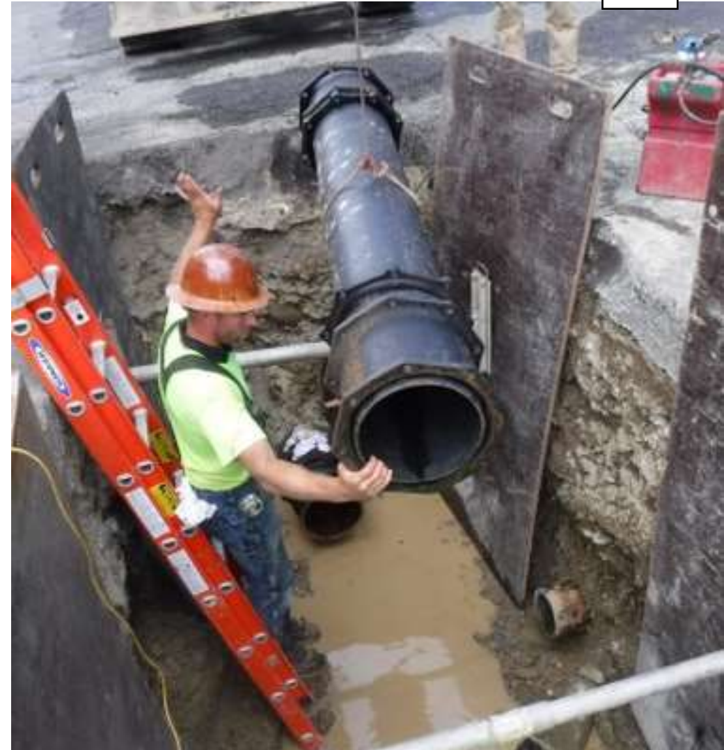
12" pipe installation
