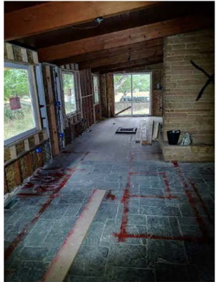
Sample interior view
