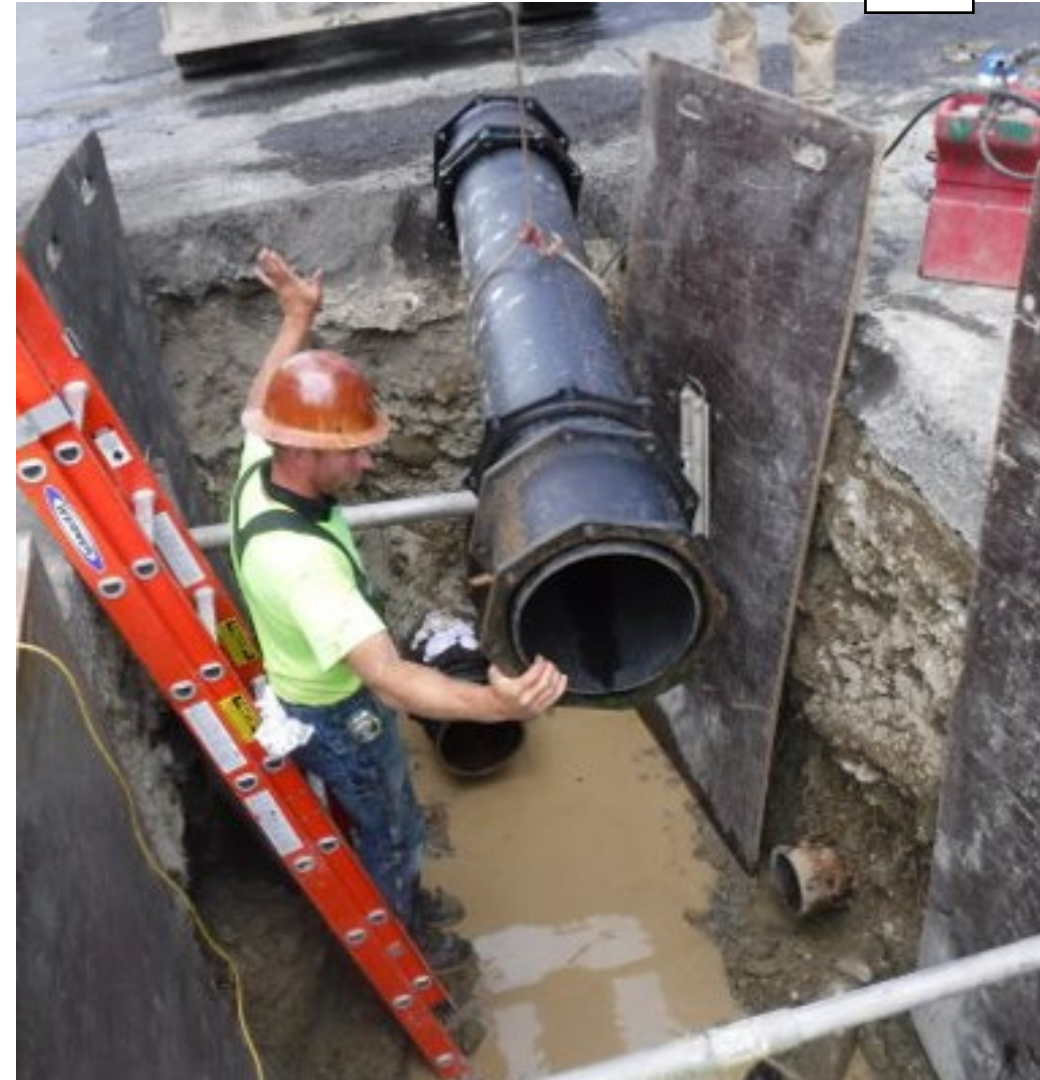
12" pipe installation
