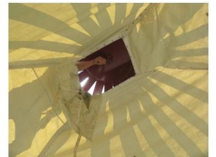
This top hole here because it is a stress point on the canvas. a separate piece covers this area.
