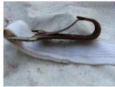
Side view of one of the hooks used to secure cover to Pergola
