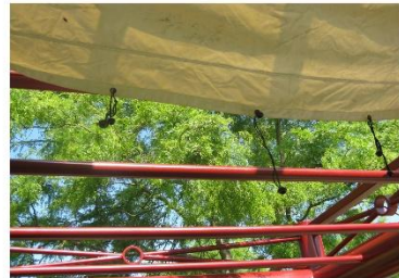
Bungees are used to further tie canvas cover around the poles of the pergola. We already have the bungees, they do not need to be included in your bid.
