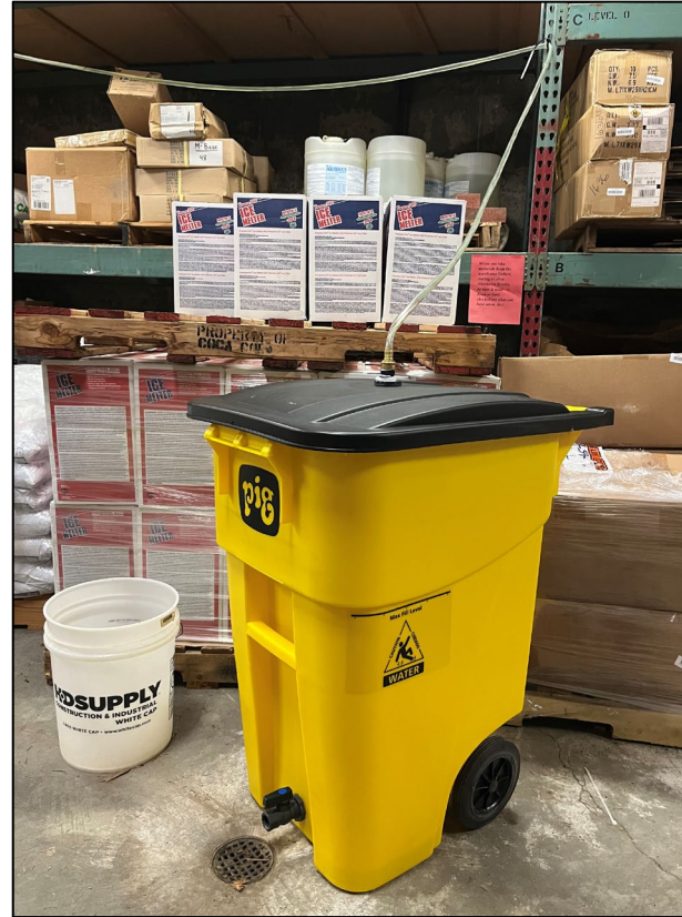
Leak collection system in warehouse
