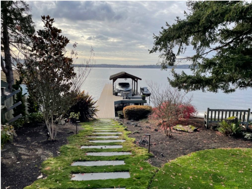
Photo 1 - Existing dock looking waterward.
