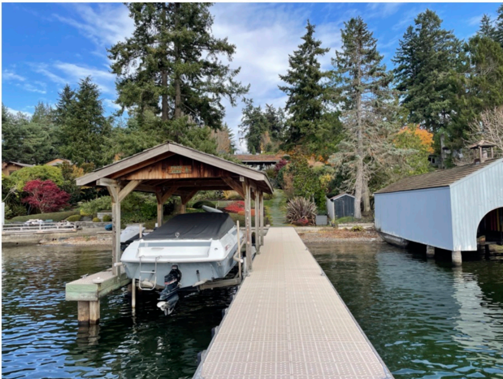
Photo 2 - Existing dock looking landward.
