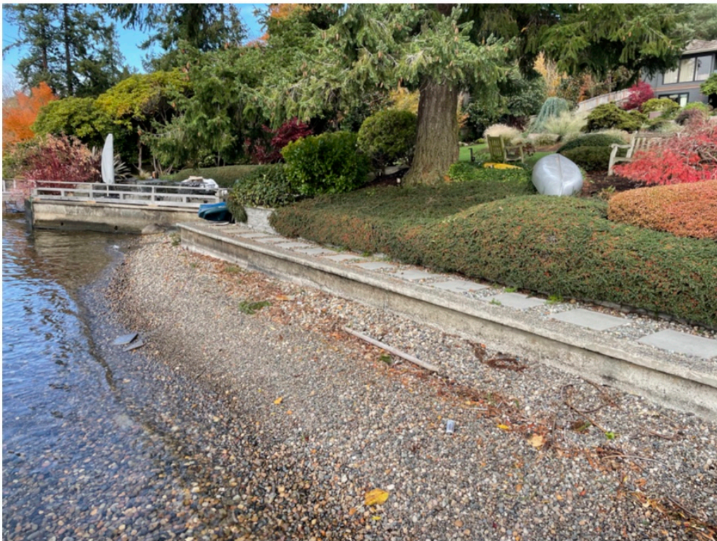
Photo 4 - Existing shoreline to the north.
