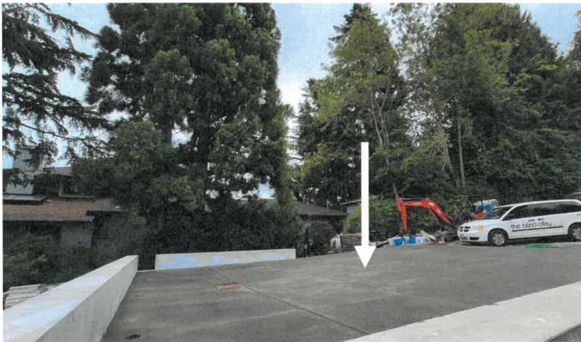
3645 Evergreen Point Rd. – One 24" Deodar cedar removed without prior consent. New driveway in location of tree (arrow). No tree protection around preserved trees as recommended by project arborist and shown in application. Revision of Administrative Tree Activity Permit application requested prior to approval.
