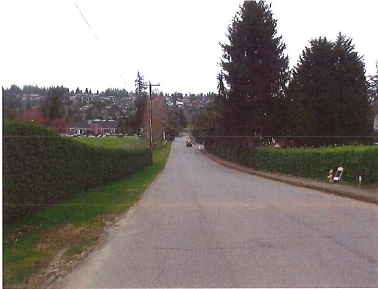
LOOKING EAST ON NE 16 TH STREET – SUBJECT RIGHT OF WAY IN DISTANT BACKGROUND
