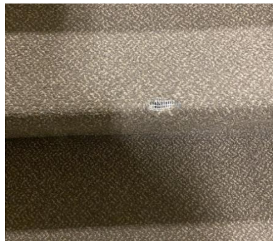
Stairs - Upper Level
