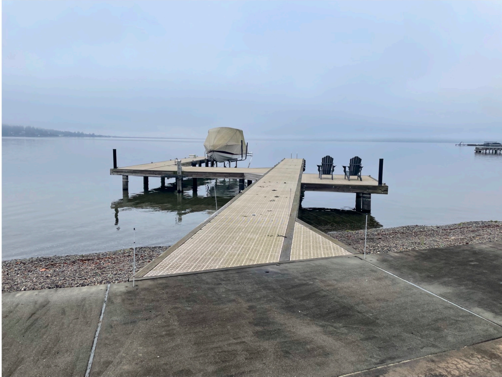
Photo 1 - Existing dock looking waterward.
