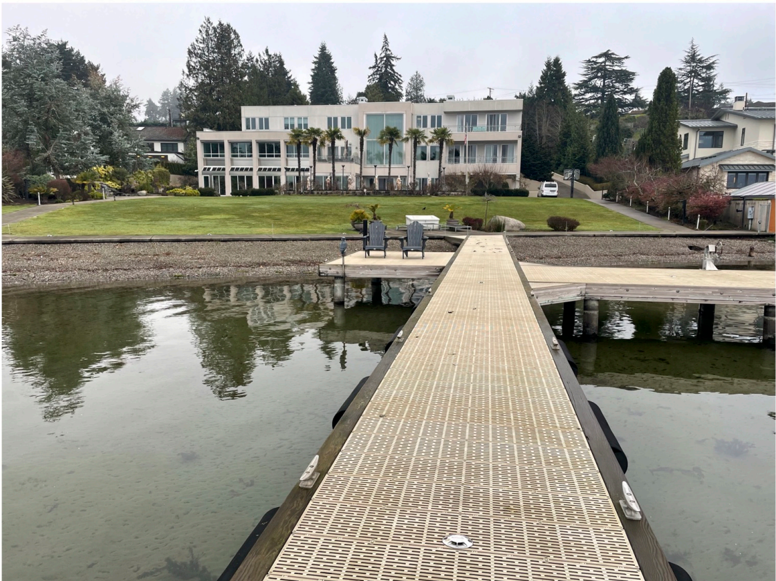
Photo 2 - Existing dock looking landward.
