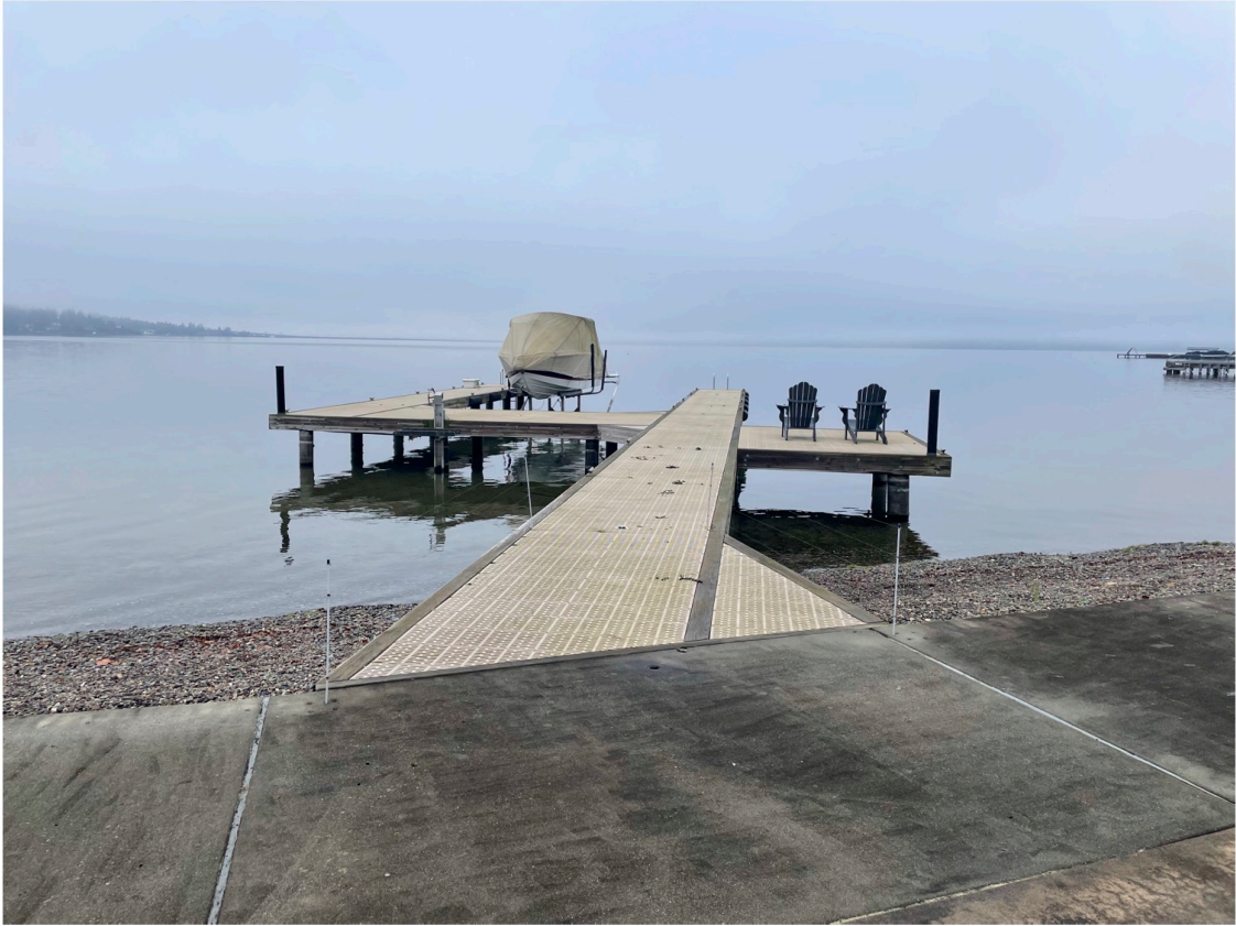
Photo 1 - Existing dock looking waterward.
