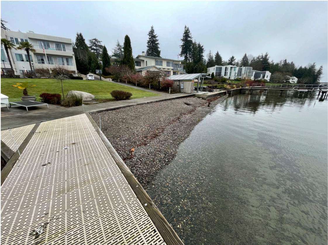
Photo 4 - Existing shoreline conditions looking south.
