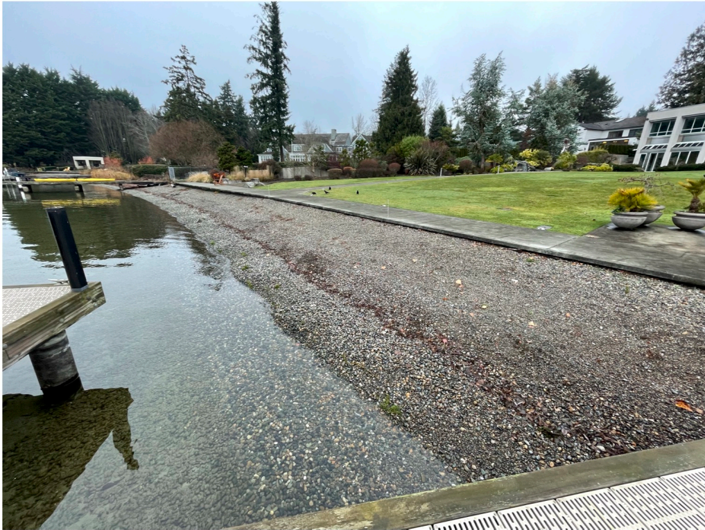
Photo 3 - Existing shoreline conditions looking north.
