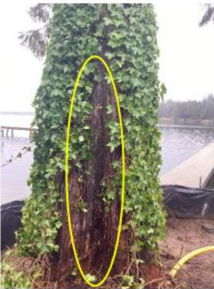
Open cavity at base of tree
