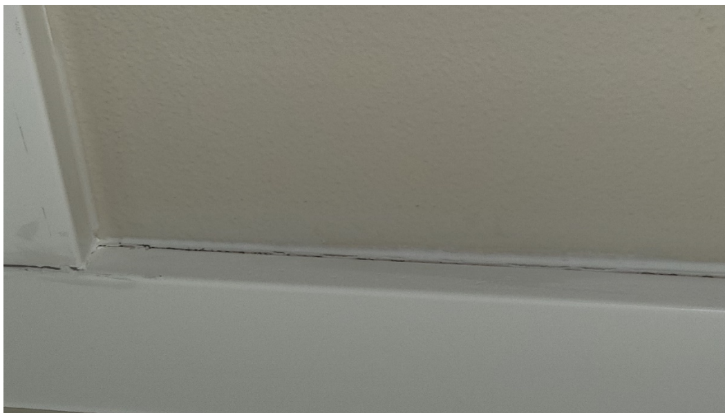
Photograph 9. Council chamber on the second floor, west wall: swollen baseboard trim, presumably from moisture impacts.
