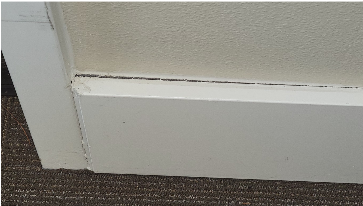
Photograph 8. Council chamber on the second floor, west wall: swollen baseboard.
