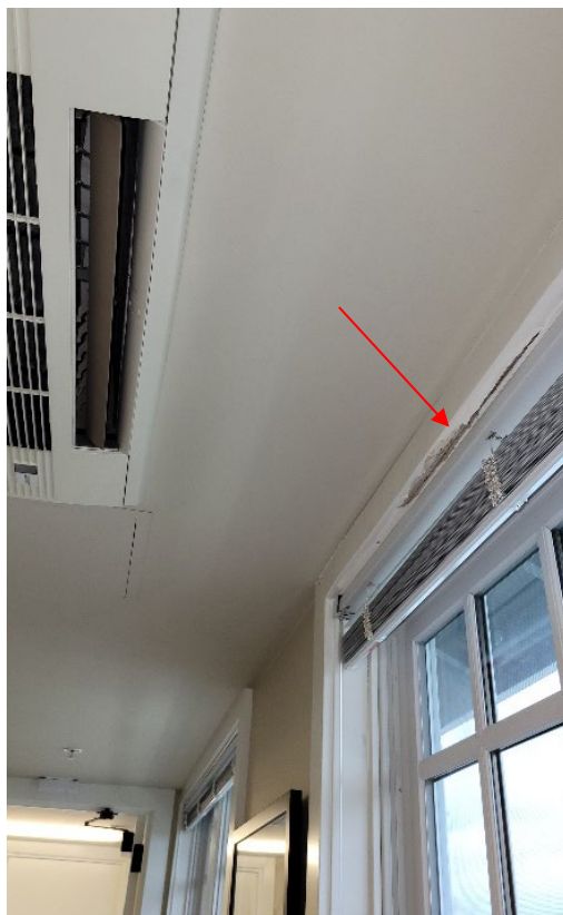
Photograph 5. Staff-only area on the second floor, north wall: delaminated paint and swollen decorative window trim.
