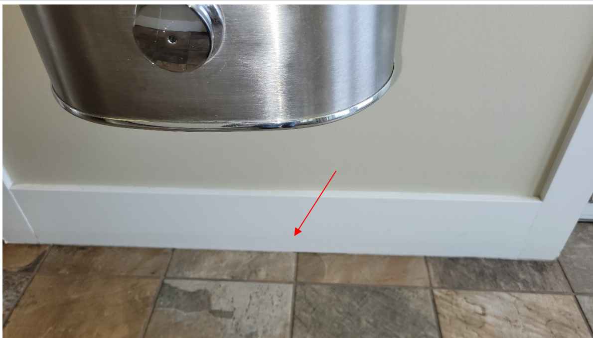
Photograph 4. Hall water cooler on the second floor: slight swelling of base board (red arrow).
